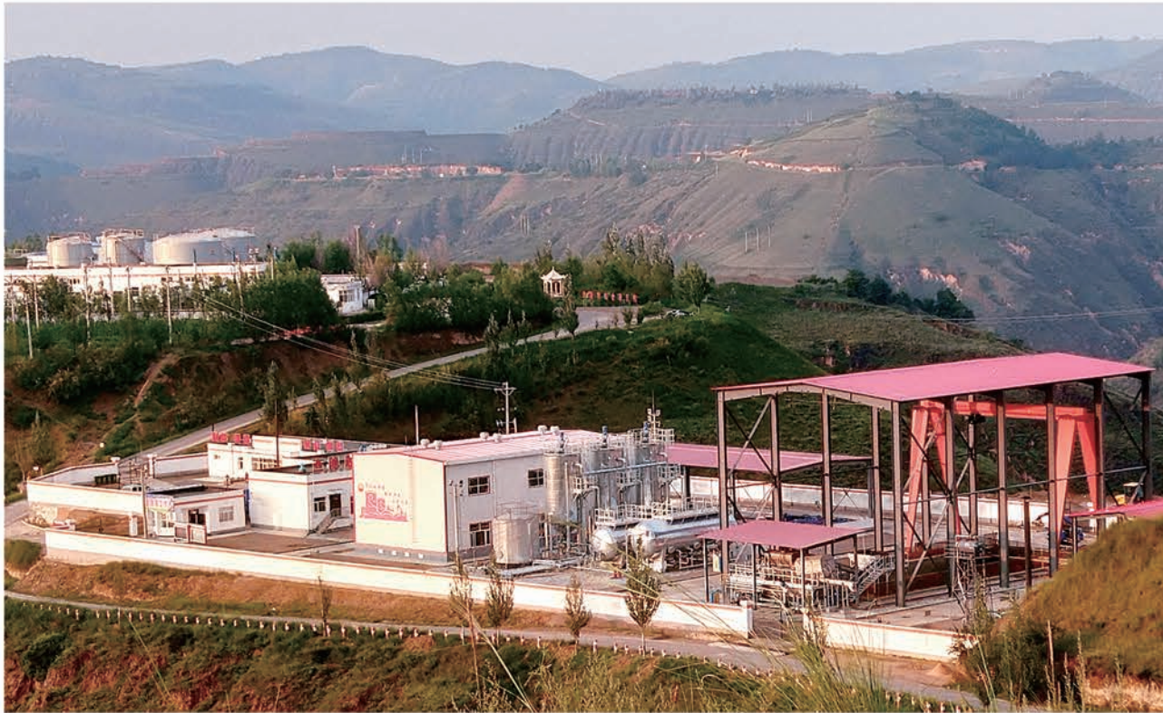
长庆油田污泥站 Sludge Station of Changqing Oilfield
