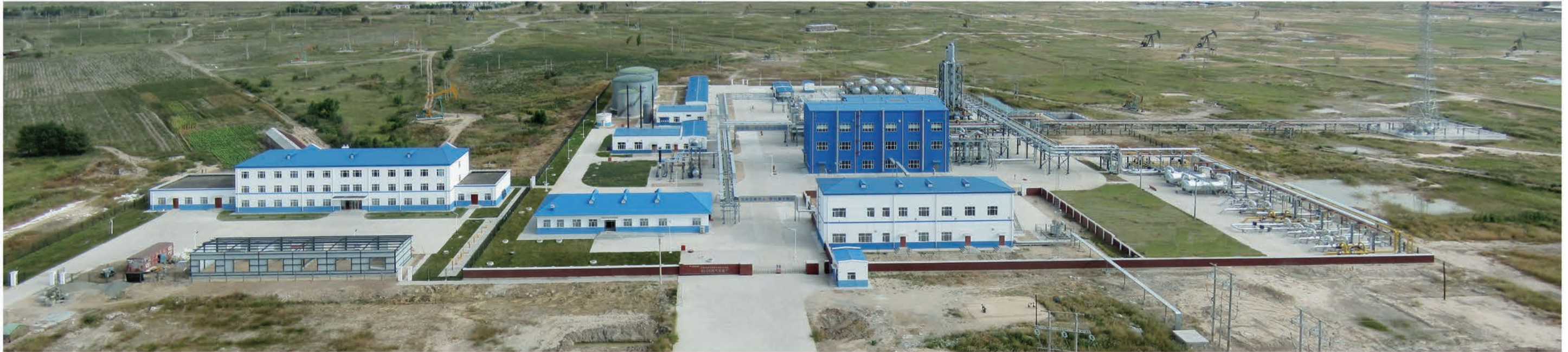
▼ 大庆油田天然气处理装置 Daqing Oilfield Natural Gas Processing Device
