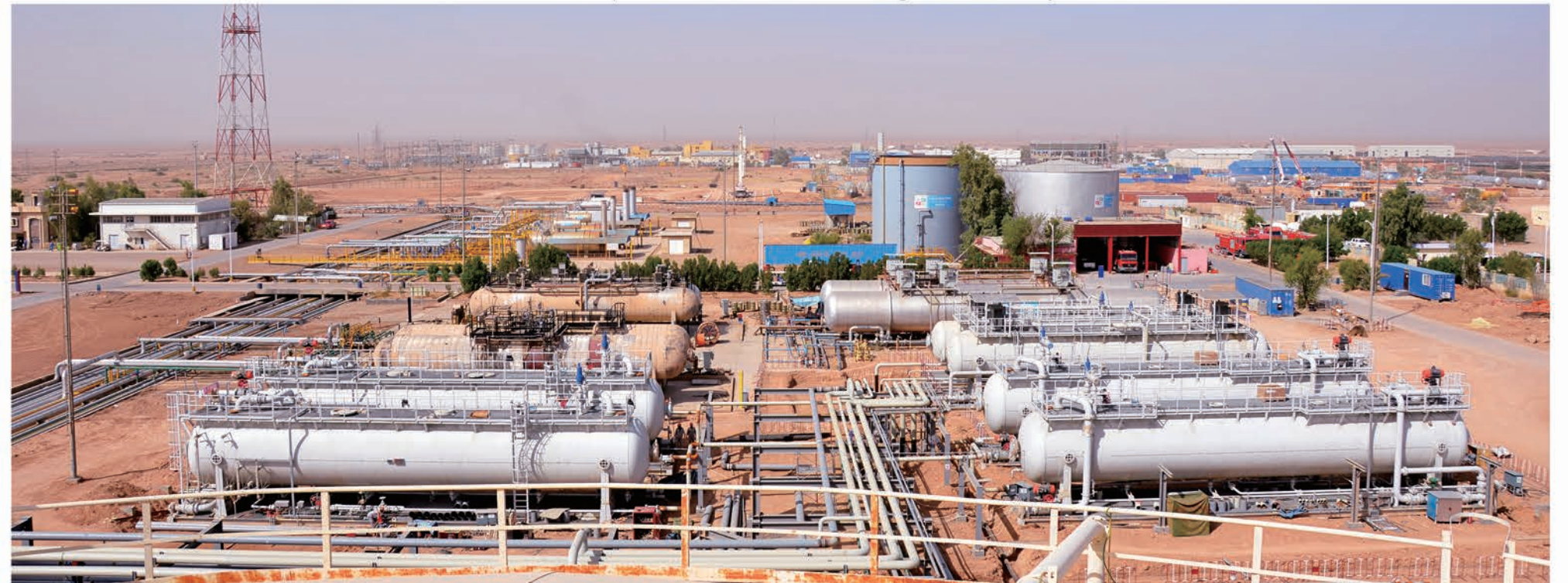
▼ 伊拉克米桑原油电脱盐改造工程 Iraq Missan Crude Oil Electro-Desalting Modification Project
