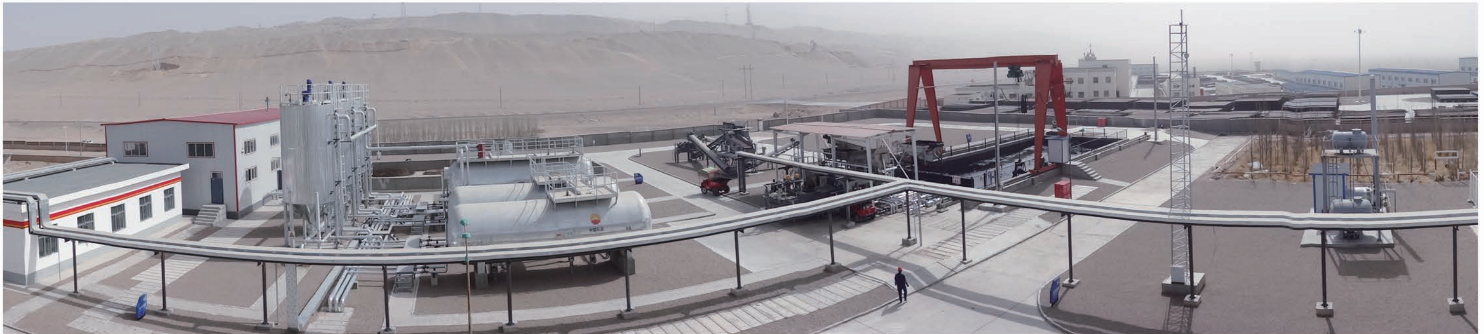
▲ 青海油田污泥处理站 Qinghai Oilfield Sludge Treatment Station
