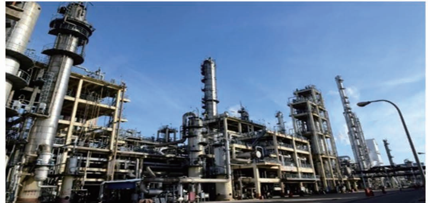
▲ 齐鲁石化百万吨级二氧化碳回收利用工程 Qilu Petrochemical's Megaton CO 2 Recovery and Utilization Project
