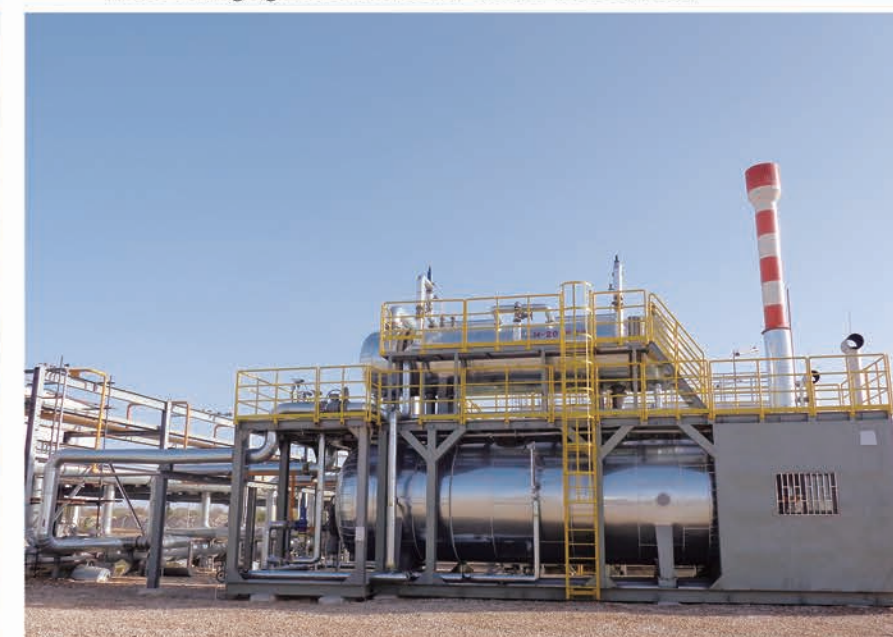
▼ 乍得BABOB油田相变式加热炉 Phase Changing Heat Furnace for Chad BABOB Oil Field
